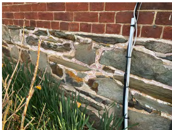
Figure 1: Ca. 1793 section- red wash on mortar joints of the foundation (left), penciling of mortar joints (right) both taken on or about April 7 and 8, 2024, by Greg Blaszc.
