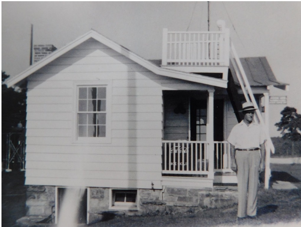
Figure 1. Terminal east side showing the observation deck and ladder stair in a ca. 1940 photo in the Ingalls Field photo collection, Hot Springs, Va. View facing west.
